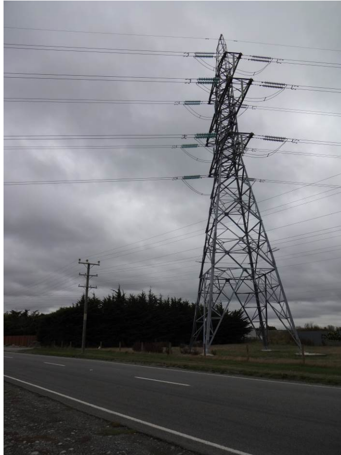
Photo 1 – Comparison of 220kV versus 33kV structures
